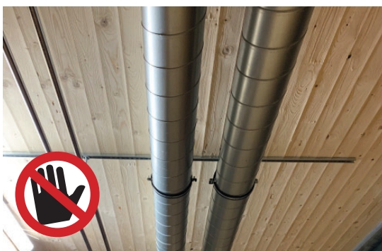
CLT ceiling subjected to excessive dampness
