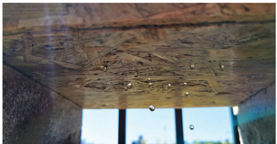
Figure 10. Water dripping through a vapour permeable Oriented Strand Board (OSB 3 type product. This is an ideal vapour permeable solution for supporting the membranes but cannot be used for waterproofing by themselves.
