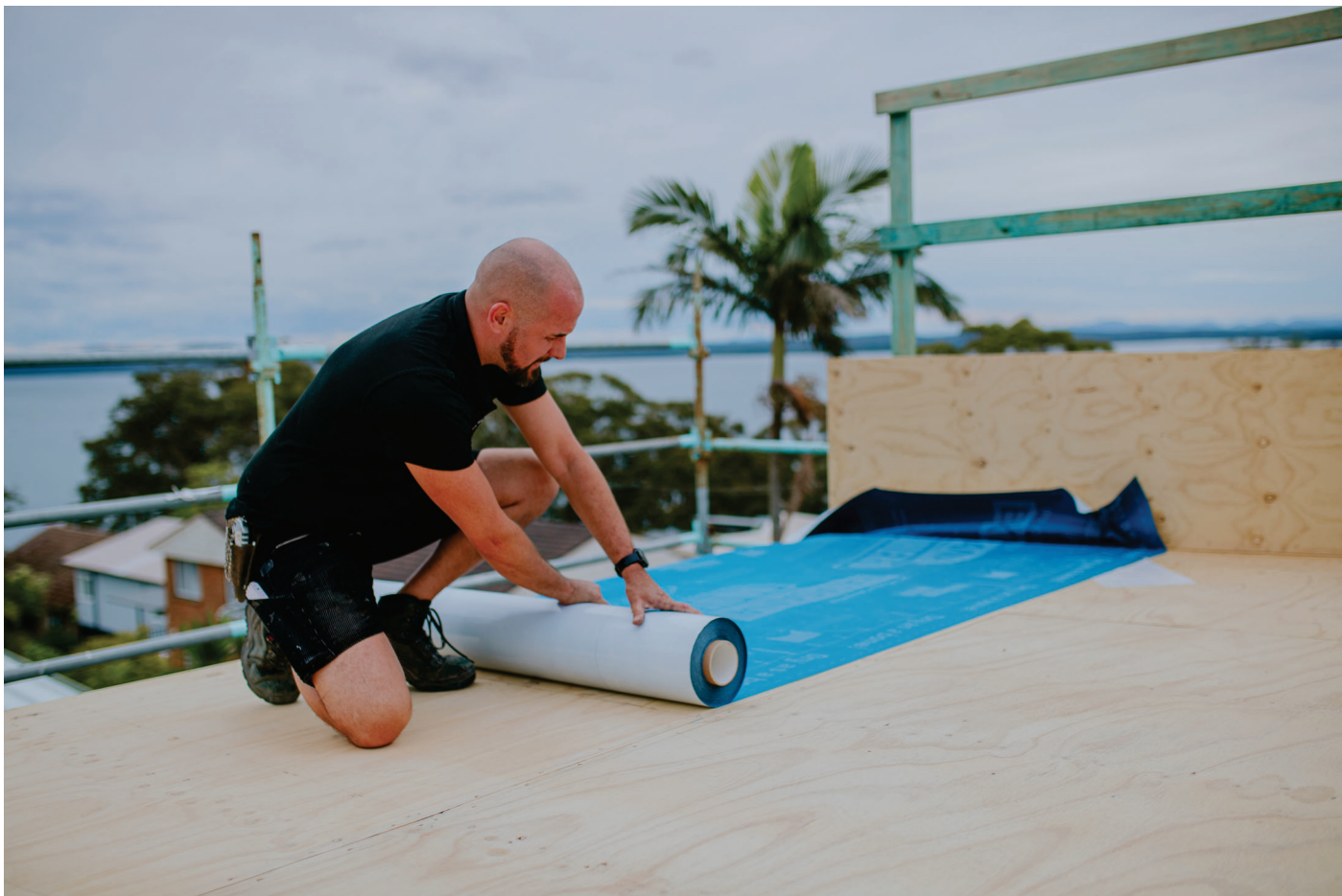
Figure 18. SOLITEX EXTASANA ADHERO application on a flat roof in Nelson Bay
