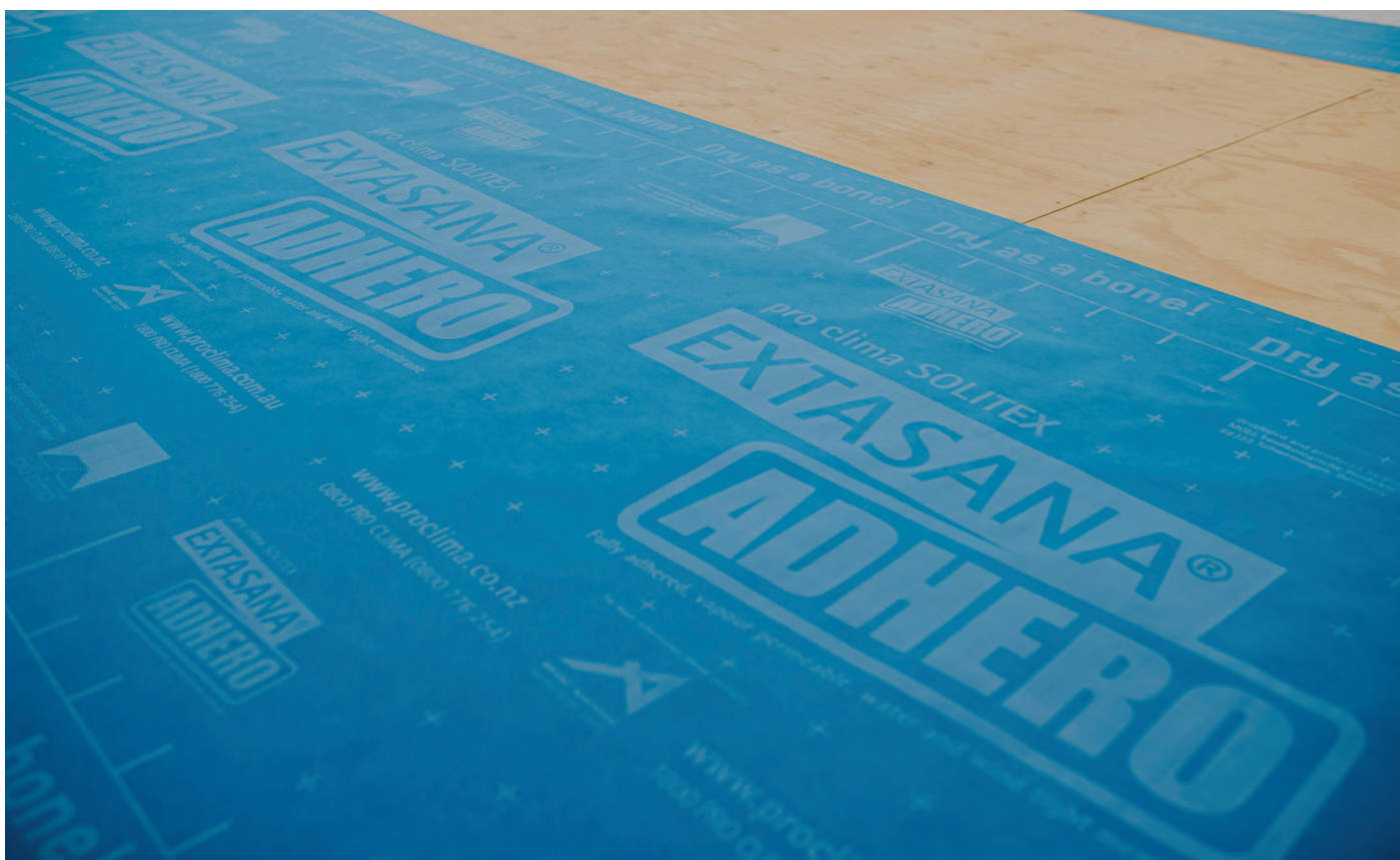
Figure 19. SOLITEX EXTASANA ADHERO on a flat roof in Nelson Bay
