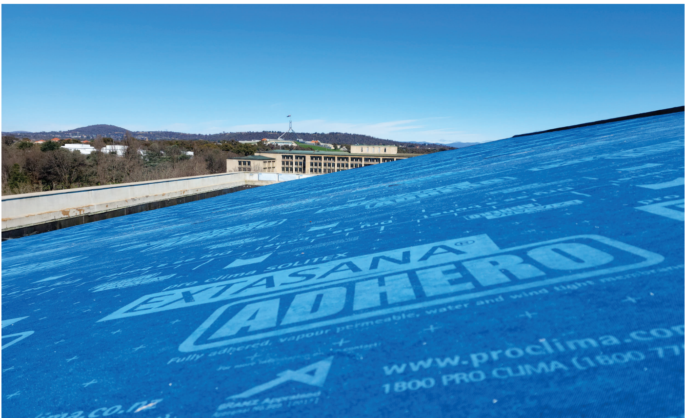
Figure 17. pro clima SOLITEX EXTASANA ADHERO on the roof of the Australian National Library
