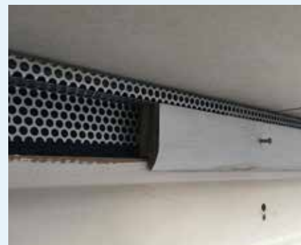
Figure 10.21: Outlets at the top of the wall with bottom vents provides a fully ventilated cladding assembly.
