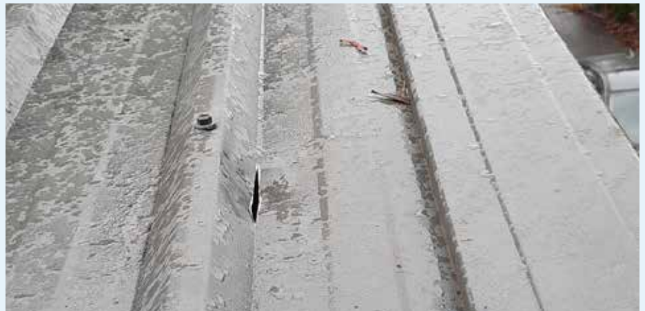
Figure 7.14: Tear in metal sheet roofing from hail damage allowing for water penetration [83]
