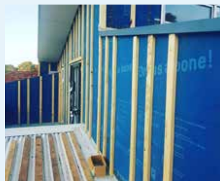
Figure 10.60: Flashing from roof to upper walls. Photo courtesy of Enduro Builders
