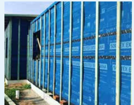
Figure 10.12: Vertical wall battens (min. 20 mm) facilitate drainage and ventilation. Photo courtesy of Craft Building Pty Ltd
