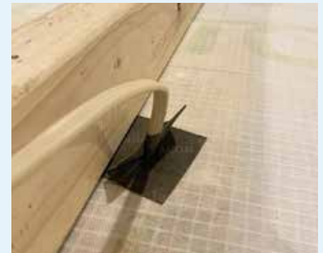
Figure 10.87: Sealing flat cables using TESCON® tapes.
