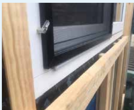
Figure 10.29: Flush window sealed with TESCON EXTORA®.
