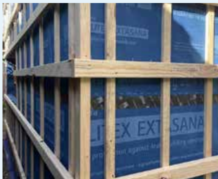
Figure 10.13: Horizontal battens fixed over vertical drainage battens. Photo courtesy of Carland Constructions Pty Ltd
