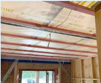
Figure 10.86: Battens perpendicular to structure.
