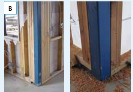
Figure 9.6: Insulate steel beams on at least one side, preferably on the outside
