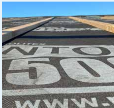
Figure 7.59: With purpose-built cavity the counter battens define the ventilation cross-sectional area. Figure 7.60: Test roof At Oakridge National Laboratory [86]
