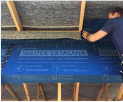
Figure 10.41: Windtight details at eaves. Photo courtesy of Passive House Construction Products (TAS) Pty Ltd
