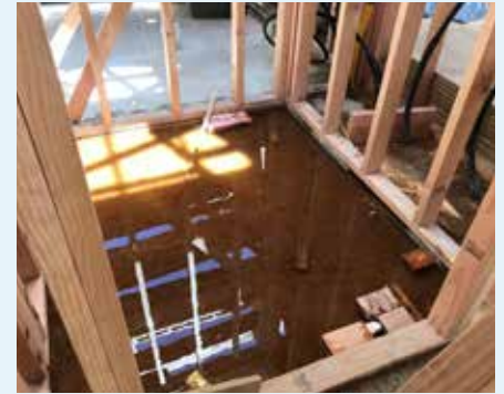
Figure 10.9: Framing should be protected from rain and below 18 % moisture content by mass [M-%].
