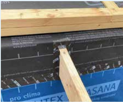
Figure 10.43: Connection of roof WRB into wall WRB. Photo courtesy of Passive House Construction Products (VIC) Pty Ltd
