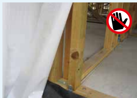
Figure 9.3: Typical uninsulated internal wall to exterior wall junctions.
