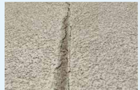
Figure 4.2: Image of failed caulking joint. Caulking cannot be relied upon for a permanently waterproof cladding system this was one of the main contributors to the Canadian condo crisis. The first line of defence is subject to temperature fluctuations (<0 to 100 °C) as well as UV. Degradation and eventual failure is certain. [51]
