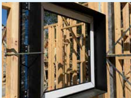
Figure 10.33: Pre-fitted window ready to accept WRB connection. Photo Courtesy of Sanctum Homes
