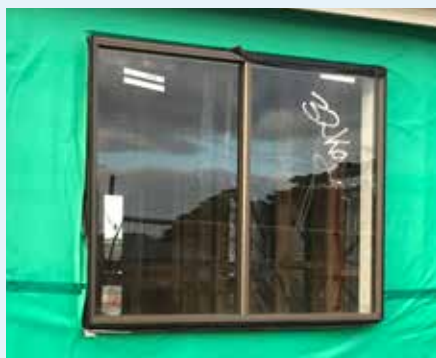
Figure 4.6: Poorly installed membranes with no connection between the window and the WRB system provide a pathway for water ingress.
