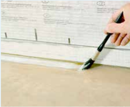
Figure 10.71: Apply primer to stabilize the surface
