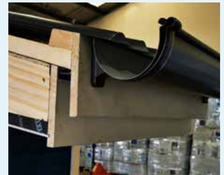
Figure 10.46: Double fascia with ventilation & drainage gap. Photo courtesy of Eclipse Passive House Pty Ltd
