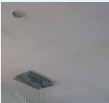
Figure 7.47: Mould growth on ceiling in Cairns from humid air reaching the back surface of the cooled plasterboard ceiling [97]
