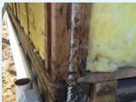
Figure 4.21: Vapour barriers can trap moisture on the cold external side of a construction system. Although this may appear to be a water leak it is actually the long term accumulation of water vapour attracted to the coldest surface. Clearly identifiable is the damage to the timber on the outer side of the studwork but not on the inside (warm side). [55]
