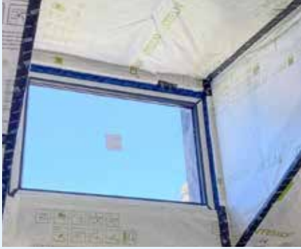
Figure 10.70: Well implemented INTELLLO® PLUS IAB connections in dormer. Photo courtesy of I-Smart Building Group
