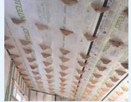
Figure 10.85: Innovative craft solution for service cavity.
