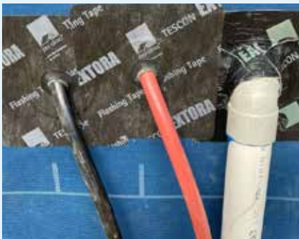
Figure 10.19: ROFLEX or TESCON EXTOSSEAL® used to seal pipe penetration.
