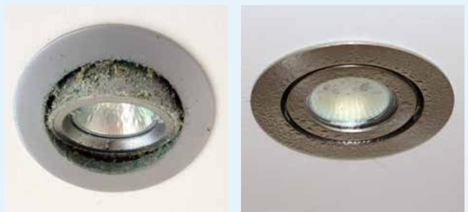
Figure 7.37: Cold surfaces and moisture laden airflow lead to condensation and fungal growth. [91]
