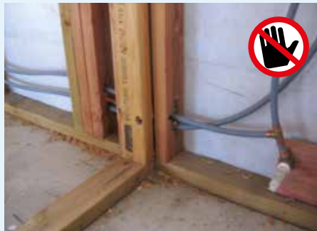
Figure 9.4: Typically insulation and services compete for space.
