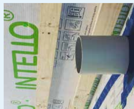
Figure 10.92: Larger ROFLEX grommets for large pipes.
