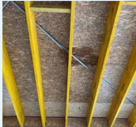
Figure 7.50: Leakage of water through fixing penetrations prior to cladding when TESCON® NAIDECK nail sealing tape was not used [98]
