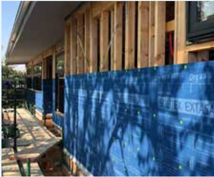
Figure 10.15: Temporary fixings for brick veneer.
