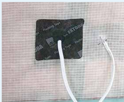
Figure 10.89: KAFLEX applied before cable connections are made.
