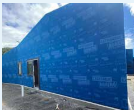
Figure 10.23: SOLITEX EXTASANA ADHERO® over rigid substrates behind architectural cladding. Photo courtesy of Scholten Group
