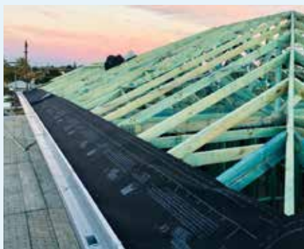
Figure 10.47: Pre-planning to drain behind metal fascia.
