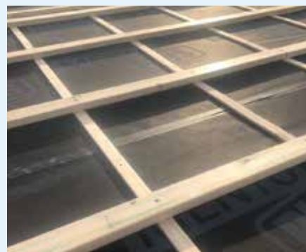
Figure 10.36: Low pitch roofing. Photo courtesy of Sanford Build Co Pty Ltd
