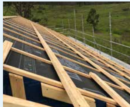
Figure 10.40: Batten size and cantilevered eaves. Photo Courtesy of Evan Graham master Builder Pty Ltd
