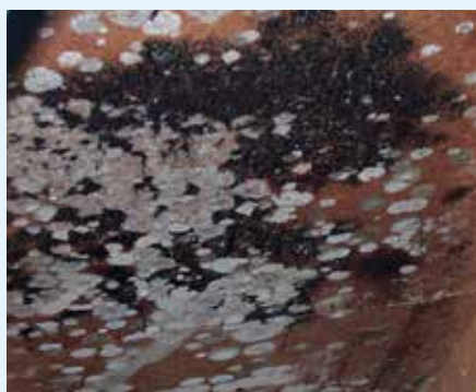
Figure 1.3: Mould in the building structure; Constructions that are not airtight do not only result in mould on the inner surfaces of structural components, but also in mould within the construction.
