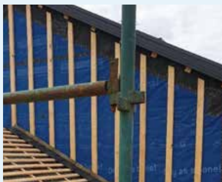
Figure 10.59: WRB as drainage layer at roof to wall connections. Photo courtesy of Passive House Construction Products Voctoria
