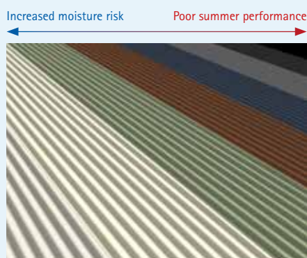
Figure 10.8: Colour of roof or wall cladding affects the hygrothermal balance.
