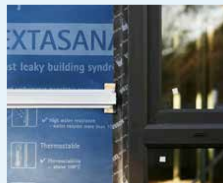
Figure 10.30: Proud window sealed with TESCON EXTORA® PROFIL.
