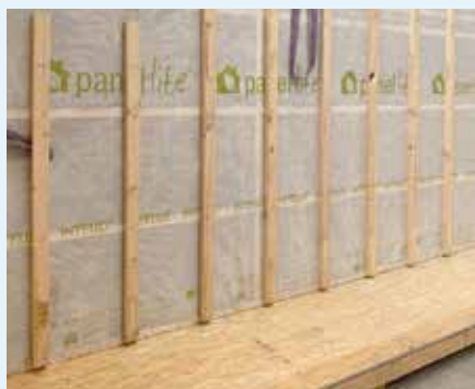
Figure 10.103: Battens configuration designed into panels. Photo courtesy of Carbonlite
