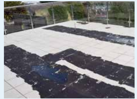
Figure 7.81: Damage to a flat roof construction due to poor waterproofing and internal water vapour management [118]
