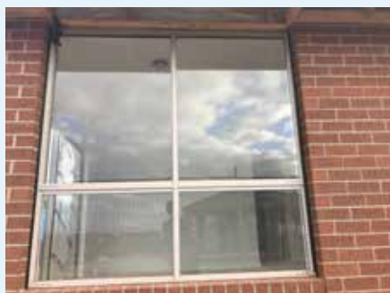
Figure 4.4: Interfaces between the cladding material and built-in components are often abutted and not sealed. This will leak when rain and wind are present. [53]
