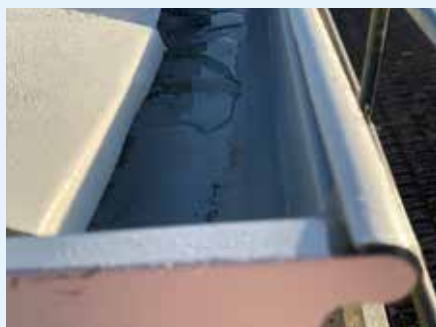
Figure 7.24: Early hours of the morning condensation due to night sky cooling [87]
