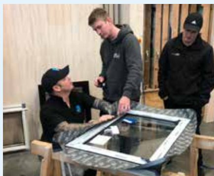
Figure 10.27: Applying CONTEGA® EXO.
