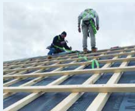
Figure 10.38: Larger batten size. Photo courtesy of Our FabHaus Pty Ltd
