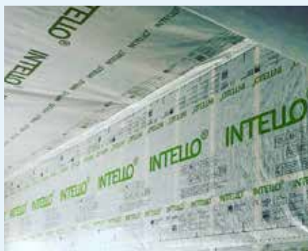
Figure 10.93: INTELLO® PLUS laid such that overlaps not in vertice.
