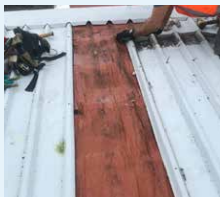
Figure 7.11: This is not a leaky roof. The amount of condensation forming on the underside of roofing metal is more than what can be absorbed or drained by the underlay and puddles form. The extreme conditions under the metal have also caused wrinkles & sagging, plus mould is starting to grow. [78]
