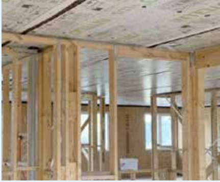
Figure 10.97: INTELLO® PLUS before non-structural partitions. Photo courtesy of Passive House Construction Products Victoria
