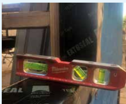
Figure 10.25: Sloped sill trimmer to shed water outwards on the surface of the TESCON EXTOSEAL®.
