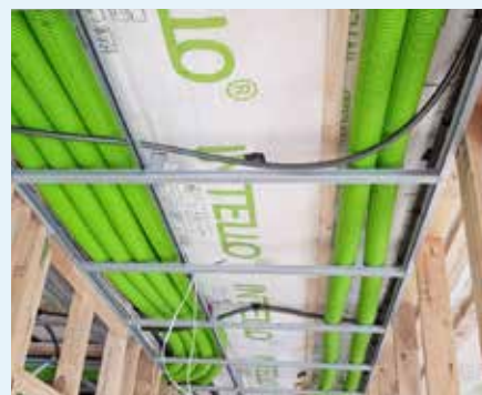
Figure 10.80: Metal feet brackets hold INTELLO® PLUS and provide rail mounting for drop ceiling.
