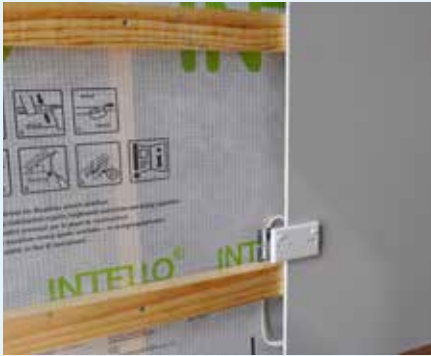
Figure 10.73: Horizontal battens for the service cavity
