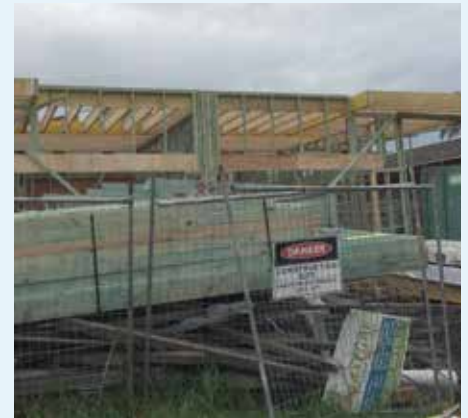
Figure 7.51: Framing timber is often allowed to get saturated on building sites before buildings are properly closed in and protected from weather [99]
