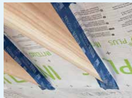
Figure 10.96: TESCON® VANA taping around structural elements.
