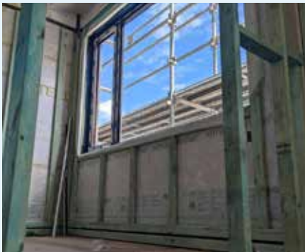
Figure 10.75: Dedicated skirting board mount timber and cable channel. Photo courtesy of Blaise Building Services
