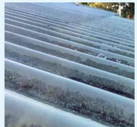
Figure 7.54: Over time the absorptivity of the roof will increase as the roof ages, surfaces dull and dirt, grime & lichens accumulate [103]
