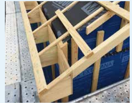
Figure 10.44: Outriggers or "attached eaves". Photo courtesy of Evan Graham Master Builder Pty Ltd
