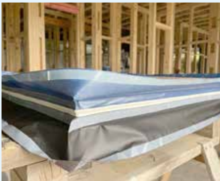
Figure 10.99: CONTEGA® IQ installed in combination with CONTEGA® EXO. Photo courtesy of Compound
