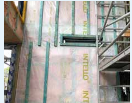
Figure 10.76: Creative battening allows for cable pathway. Photo courtesy of Blaise Building Services
