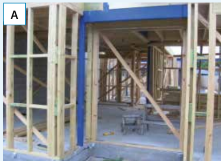
Figure 9.6: Insulate steel beams on at least one side, preferably on the outside
