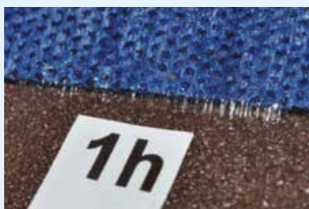
Figure 4.4: Interfaces between the cladding material and built-in components are often abutted and not sealed. This will leak when rain and wind are present. [53]
