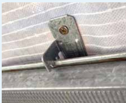
Figure 10.81: Furring channel & clip over INTELLO® PLUS
