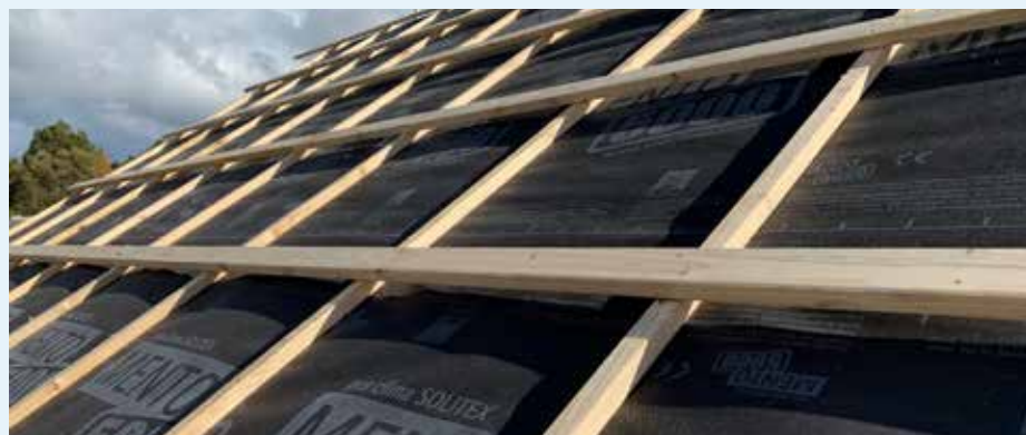
Figure 7.18: Ready for the roofing cladding to be installed, this site shows the arrangement of counter battens (running vertically) and battens (running horizontally) to form a drained and ventilated cavity. *Specific products may vary. [84]
