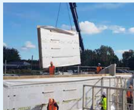
Figure 10.104: Panelised systems craned on site. Photo courtesy of pro clima NZ
