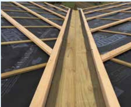
Figure 10.56: WRB continuous under valley boards. Photo courtesy of Passive House Construction Products Victoria
