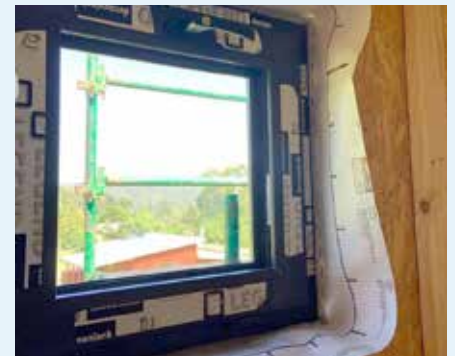
Figure 10.100: Pre-installed INTELLO® PLUS strip to window prior to install. Photo courtesy of Ben Amor
