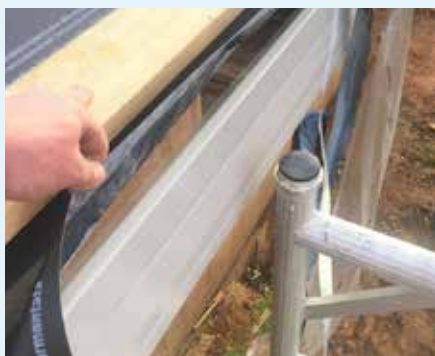
Figure 10.49: Bonding membrane to metal fascia.
