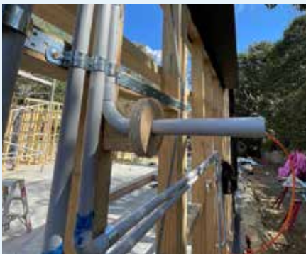
Figure 10.17: Prior planning for fixing of membrane around penetration.
