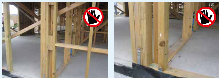
Figure 9.2: Typical uninsulated corners.
