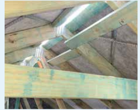
Figure 10.54: Gap in WRB at ridge to ventilate the attic. Photo courtesy of TruLine Construction
