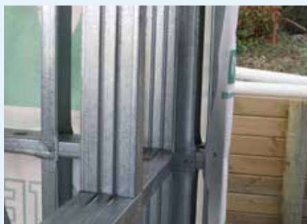
Figure 9.7: Insulate steel structures on at least one side preferably on the outside
