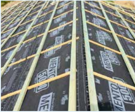
Figure 10.53: Membrane over ridge. Photo courtesy of I-Smart Building Group
