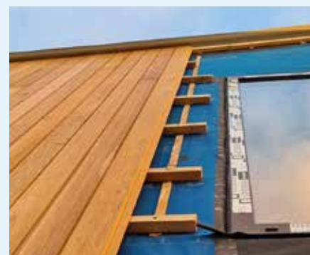
Figure 10.32: Batten position allows for CONTEGA® EXO connection.
