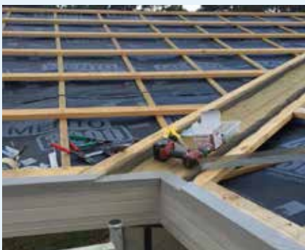
Figure 10.58: Counter batten system and fascia height. Photo courtesy of Passive House Construction Products Victoria
