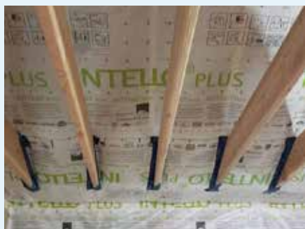
Figure 10.95: Structural penetrations of INTELLO® PLUS.
