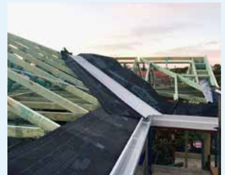
Figure 10.57: WRB continuous under valley trays. Photo courtesy of I-Smart Building Group
