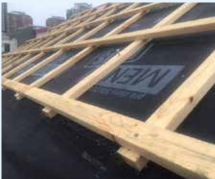
Figure 10.45: Allowing for ventilation inlet at eave. Photo courtesy of Eclipse Passive House Pty Ltd
