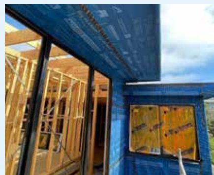
Figure 10.62: Wrapping eaves. Passive House Construction Products Victoria
