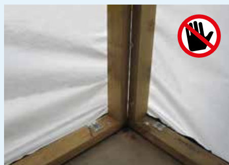
Figure 9.2: Typical uninsulated corners.
