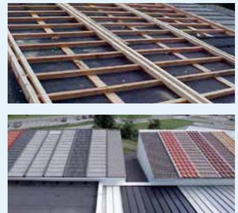
Figure 7.59: With purpose-built cavity the counter battens define the ventilation cross-sectional area. Figure 7.60: Test roof At Oakridge National Laboratory [86]
