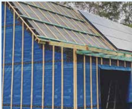
Figure 10.11: Drainage battens applied vertically. Photo courtesy of Lou Projects.
