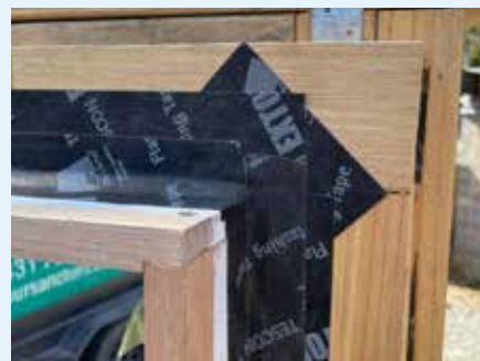
Figure 10.34: TESCON EXTORA® seal to the window reveal. Photo Courtesy of Sanctum Homes
