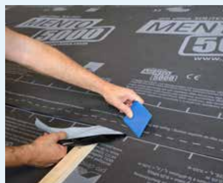
Figure 10.64: SOLITEX MENTO® connect self-adhesive zones
