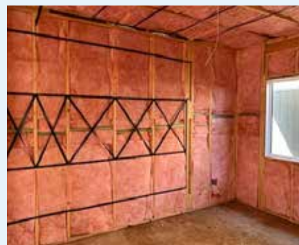
Figure 10.82: Plastic packaging strap used to hold wall/ceiling insulation.
