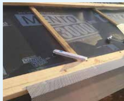
Figure 10.50: Vermin mesh and UV protection. Photo courtesy of Passive House Construction Products (TAS) Pty Ltd
