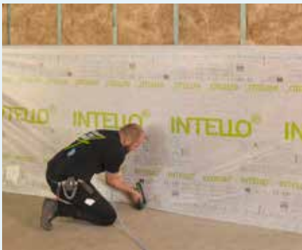
Figure 10.68: Installation of INTELLO® PLUS at wall sections
