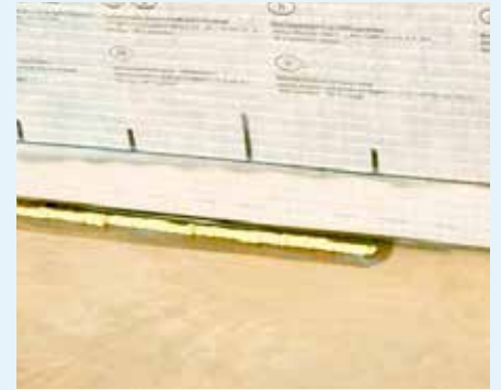
Figure 10.72: : Use ORCON® CLASSIC to connect the INTELLLO® PLUS to the concrete floor.
