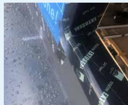
Figure 10.26: pro clima bonding technology to metal flashings.
