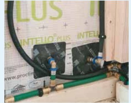
Figure 10.74: Vertical battens for the service cavity. Photo courtesy of Michael Limb Builders
