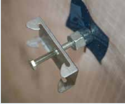
Figure 10.84: Adjustable furring channel clip with thread.
