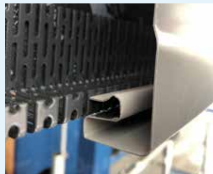
Figure 10.52: Custom made vent grille. Photo courtesy of Craft Homes Limited (NZ)
