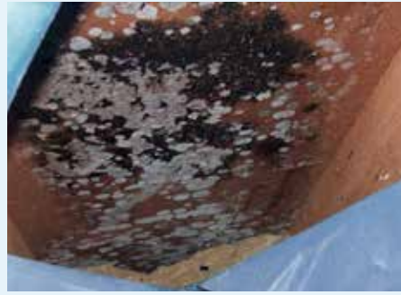
Figure 7.26: Having water on the inside of our buildings in the wrong place at the wrong time is when problems start to occur.
