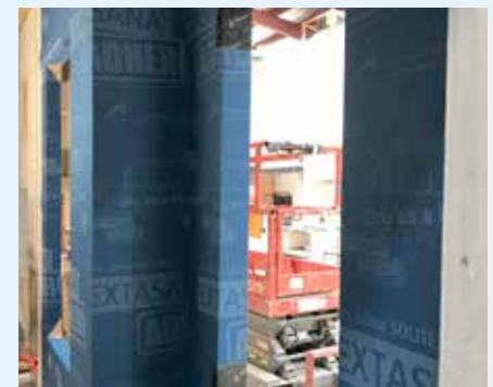
Figure 3.15: SOLITEX EXTASANA ADHERO®, full adhesive backed membrane for high pressure system weatherproofing. Façade Testing NZ Limited, Wellington, New Zealand.
