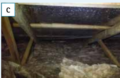
Figure 7.42: Moisture related issues on aluminium foil condensing surfaces [74]
