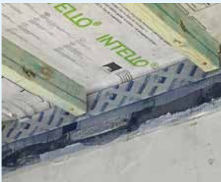
Figure 10.88: CONTEGA® PV connection to masonry.
