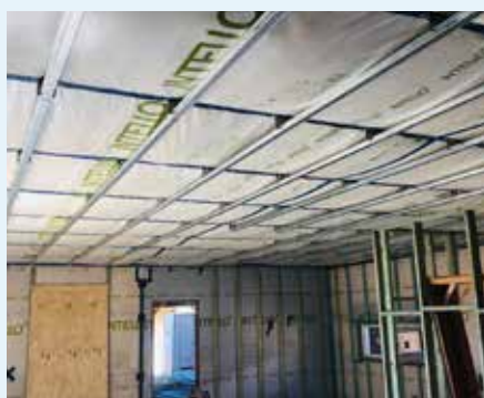
Figure 10.83: Completed INTELLO® PLUS ceiling with furring channel and clip.
