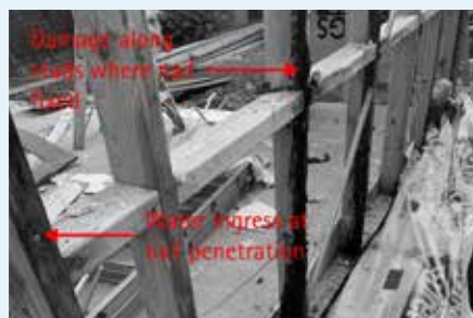
Figure 6.13: High resistance membranes provide little drying capacity and "safety buffer" for when things don't go according to plan. A site in Marrickville, Sydney, with direct fix cladding allowed water penetration through the nail fixings leading to water ingress and very limited drying potential leading to structural damage. [72]
