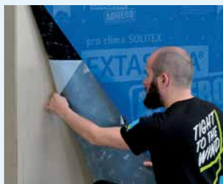
Figure 10.2: Fully adhesive membranes over rigid board
