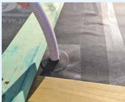
Figure 10.61: PV conduits sealed with ROFLEX 20. Photo courtesy of Truline Construction
