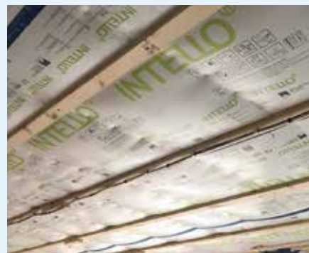
Figure 10.78: Blown-in insulation.
