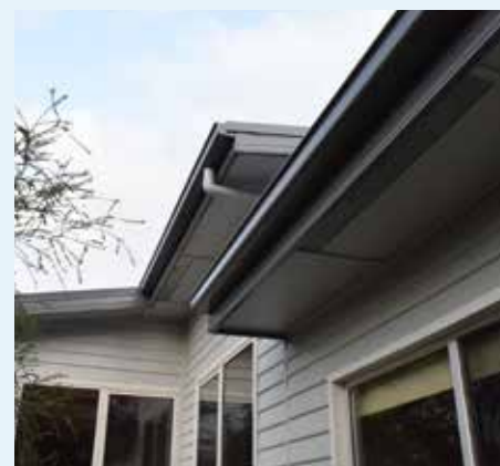
Figure 7.73: Bushfire Mesh designed into eave soffit to allow ventilation and prevent burning embers from entering as required by AS 3959 [114]
