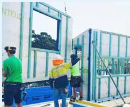
Figure 10.105: Panel connections made on site. Photo Courtesy of I-Smart Building Group
