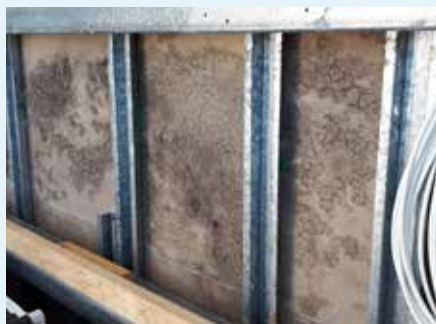
Figure 4.22: Mould growth caused by back diffusion in Mackay, Australia. [56]
