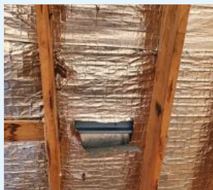
Figure 7.12: Temperature fluctuations cause expansion and contraction of underlay materials which can lead to rips and tears, especially in composite membranes where different materials behave differently with varying temperatures. [78]
