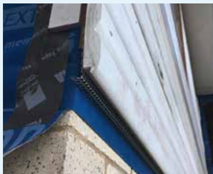
Figure 10.20: Vents at bottom of wall provide drainage and some venting of the wall cavity. Photo courtesy of Eclipse Passive House Pty Ltd
