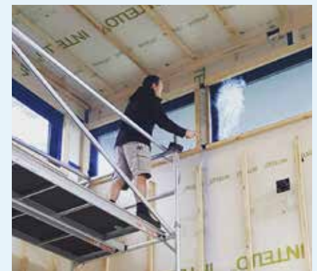
Figure 8.3: Using smoke bottle diagnostic tool to check for air leaks during Blower Door testing. Photo courtesy of Michael Limb Builders
