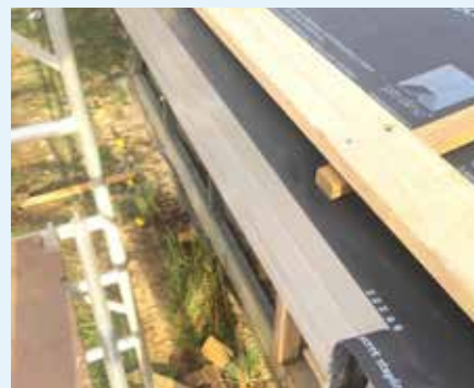
Figure 10.48: Draining over metal fascia. Photo courtesy of Passive House Construction Products (TAS) Pty Ltd
