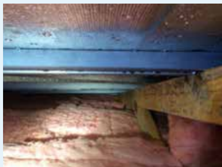
Figure 7.1: Attic space with wet foil sarking in contact with perimeter ceiling insulation [73]
