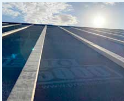
Figure 10.37: Min. 20 mm counter batten height
