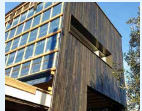
Figure 10.14: For vertical cladding horizontal battens with vertical drainage battens. Photo courtesy of Evan Graham Master Builder Pty Ltd
