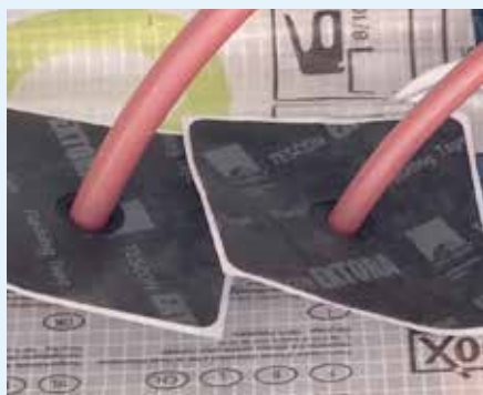
Figure 10.91: ROFLEX installed before pipe connections are made.
