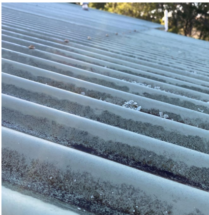
Figure 6: Over time the absorptivity of the roof will increase as the roof ages, surfaces dull and dirt, grime and lichens accumulate. (Image: Jesse Clarke, Pro Clima Australia)
