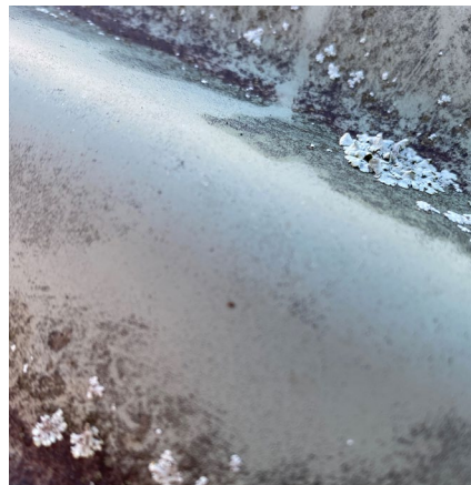
Figure 6: Over time the absorptivity of the roof will increase as the roof ages, surfaces dull and dirt, grime and lichens accumulate. (Image: Jesse Clarke, Pro Clima Australia)
