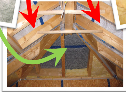
Figure 3: One roof, similar exposure, dramatically different results: non-porous SOLITEX MENTO® membrane straight ahead, on left/right faces a micro-porous membrane.
