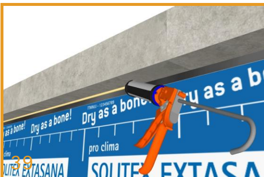
39 Seal to the Soffit Using ORCON® CLASSIC The SOLITEX EXTASANA® 30 mm overlap should be adhered to the soffit using a bead of ORCON® CLASSIC. (See matrix at step 61 for compatibility).
