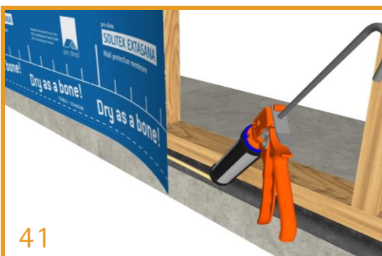
41 Seal to Damp Course Using ORCON® CLASSIC When the frame is finished flush with the slab edge, SOLITEX EXTASANA® is adhered to the damp course using ORCON® CLASSIC.
