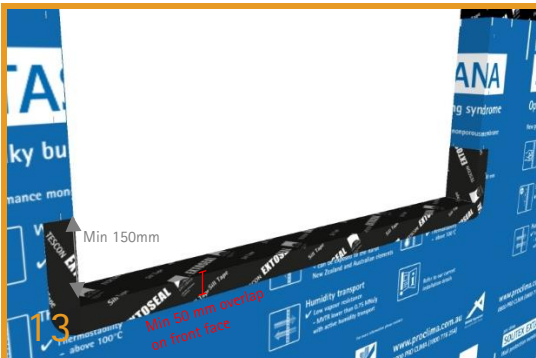
Applying TESCON EXTOSEAL® Sill Tape TESCON EXTOSEAL® Sill Tape should extend minimum 150 mm up the jambs. The corners of the TESCON EXTOSEAL® are stretched & adhered into place.
