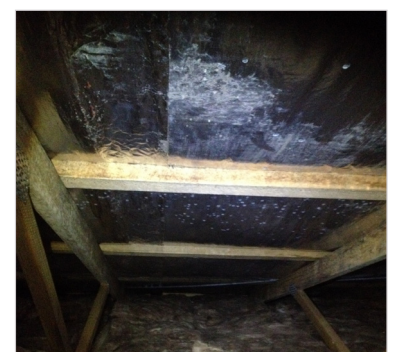
Mould growth on foil-faced blanket system. High humidity in the roof space, a inclusion of a condensing surface and the lack of moisture egress result in mould growth.
