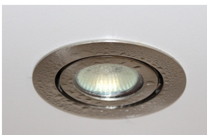
Figure 20: Cold surfaces and moisture-laden airflow lead to condensation and fungal growth.
