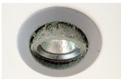
Figure 20: Cold surfaces and moisture-laden airflow lead to condensation and fungal growth.
