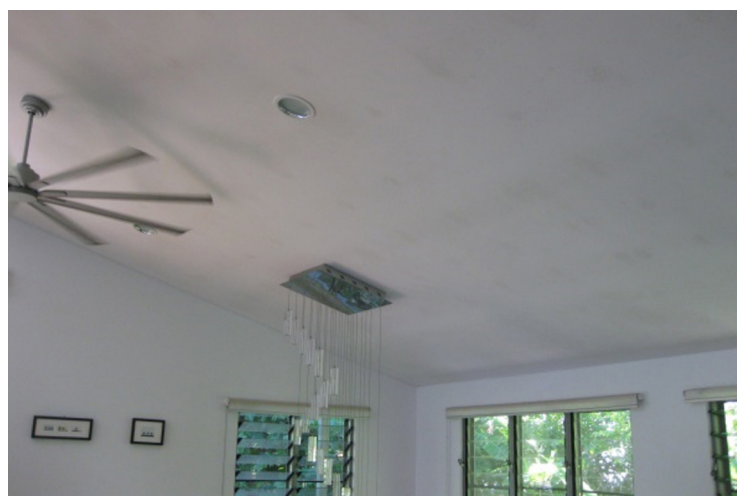
Figure 33: Mould growth on the ceiling in Cairns from humid air reaching the back surface of the cooled plasterboard ceiling. Photo courtesy: Heath Bussell, Queensland Construction and Building Commission.
