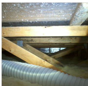
Condensation forming day and night on the inside surface of the sarking system. Mould growth on the structural elements within the roof space. A lack of vapour permeability and zero sorptive capacity on the membrane means that a perfect condensing surface is provided.
