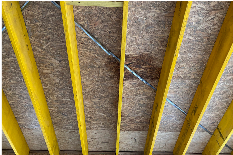
Figure 35. Leakage of water through fixing penetrations prior to cladding when TESCON® NAIDECK nail sealing tape was not used.
