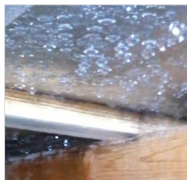
Detailed photograph of water dripping off the sarking system onto ceiling insulation. On a 23° slope roof water will start to run down a roof at 150 g/m 2 of condensate (BS 5250).
