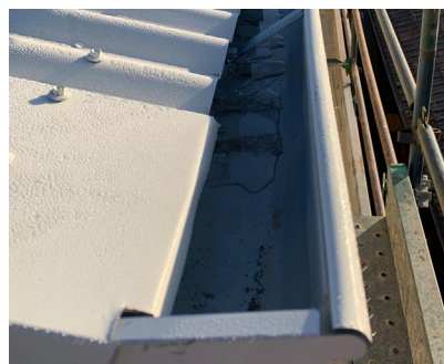
Figure 8: (left) Early hours of the morning condensation due to night-sky cooling. Wollongong, Australia Institute of Refrigeration and Heating (AIRAH) high-performance housing project, Photo Courtesy: Stephen Cuthbert, AIRAH.
