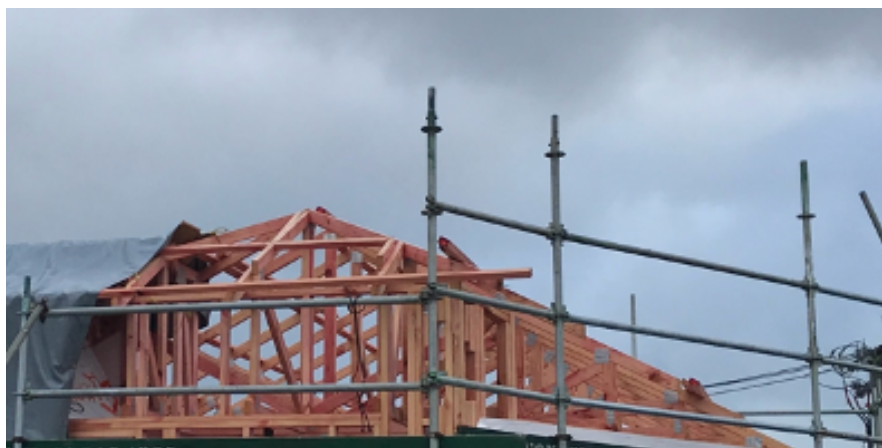
Figure 36: Framing timber is often allowed to get saturated on building sites before buildings are properly closed in and protected from the weather.
