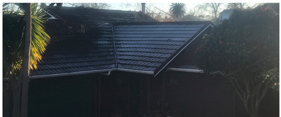
Figure 9: (below left) Night-sky radiation can reduce roof surface temperatures to below zero, causing frost, even when the ambient air temperature is above 0°C, Photo Courtesy: Matthew Cutler-Welsh, Auckland.
