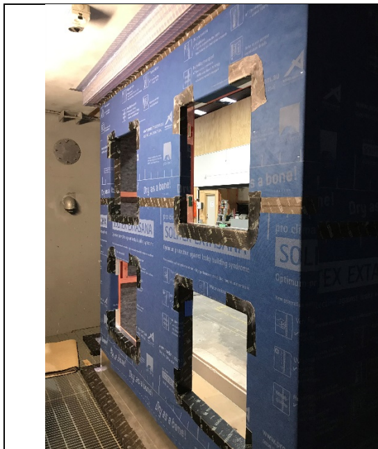
VM1 testing including pro clima SOLITEX EXTASANA®, a windtight & watertight weather resistive barrier, Helfen test laboratory, Wellington New Zealand
