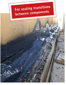
Transitions between components with different materials and with lots of edges and corners – simply spray on AEROSANA VISCONN and everything is sealed!
