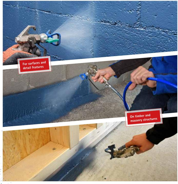
With the humidity-variable AEROSANA VISCONN spray-on or brush-on airtightness seal, you can work extremely quickly whether on surfaces such as non-plastered masonry or porous panel-form materials, or when creating joints between components on timber and masonry structures.
